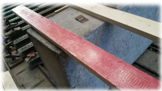
Picture 7: Spread PF glue mixture on beam
