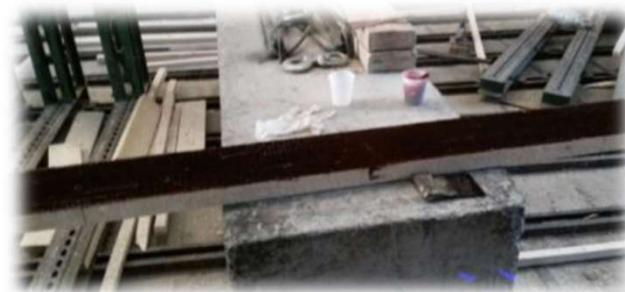
*Picture 1: Spread PFL glue mixture on beam*
